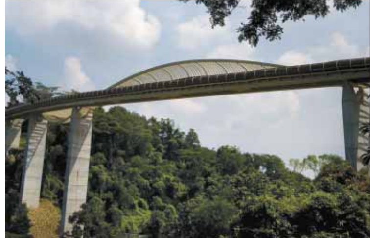
The Henderson Wave bridge is part of the Southern Ridges treetop walk
