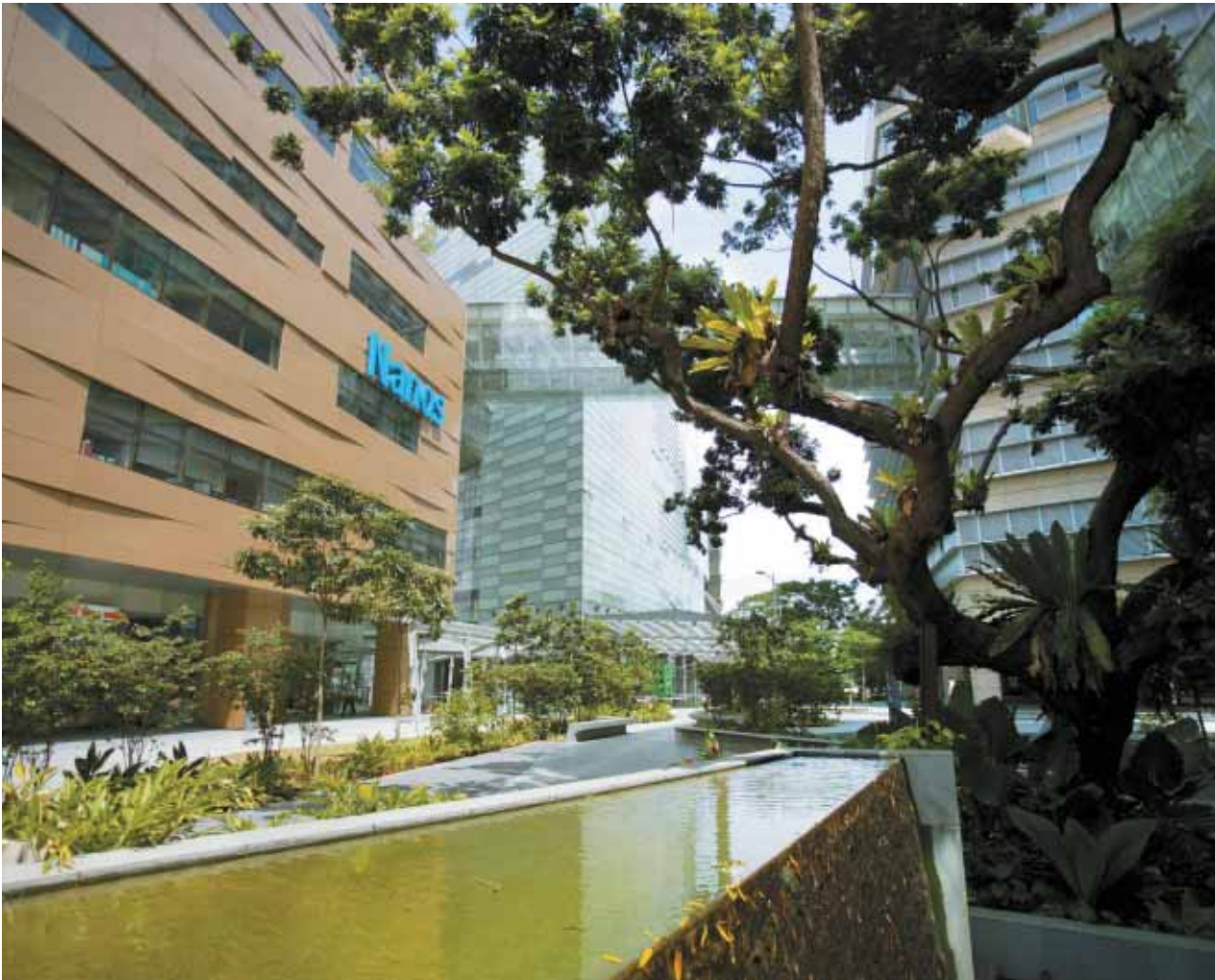
Singapore's biomedical hub, Biopolis, incorporates environmentally sustainable features like district cooling and building-integrated photovoltaics
