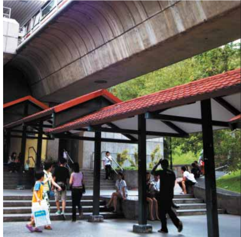
Covered linkways to MRT stations make public transport more accessible and convenient
