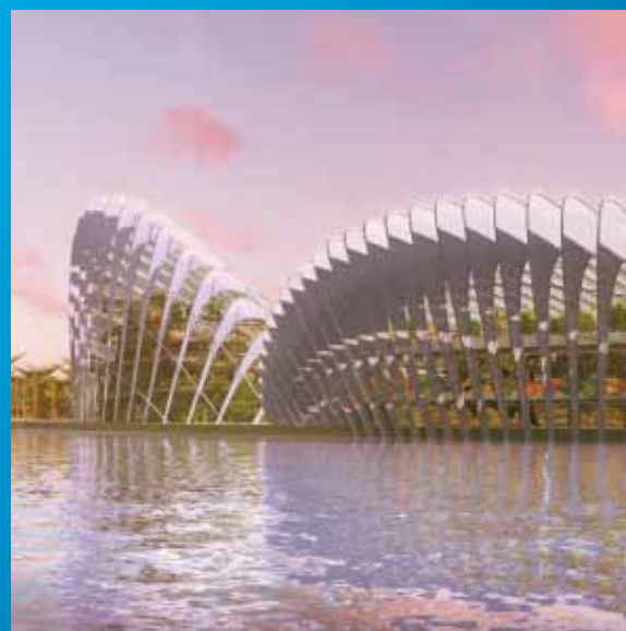
Conservatories, Gardens at Marina South
